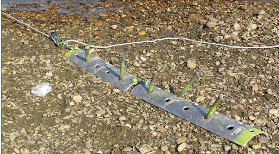
Figure 15—Two Anchor Plates Shackled Together and Fixed with Rebar
