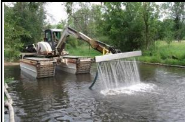
Sediment agitation with a hydraulic spray bar
