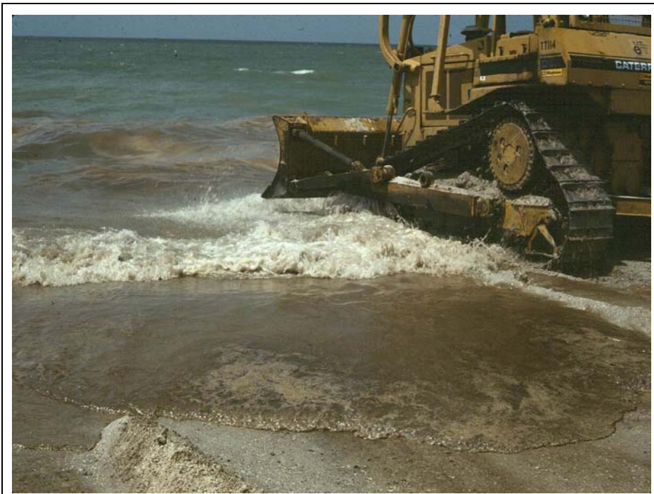
Typical brown foam observed during sediment relocation, indicating interaction between oil and fine sediments. No oil or sheen on the water is visible.
