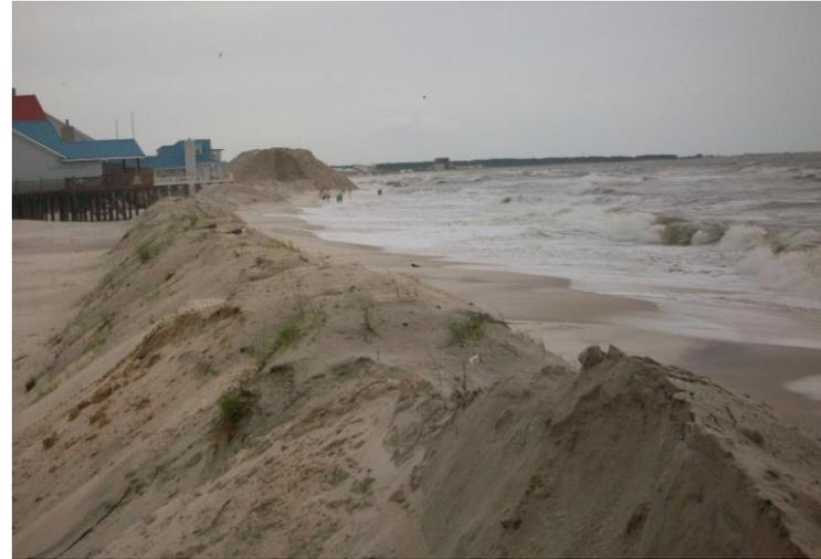
Sand ridge constructed seaward of beach houses. Note that wave uprush reaches to the toe of the ridge.
