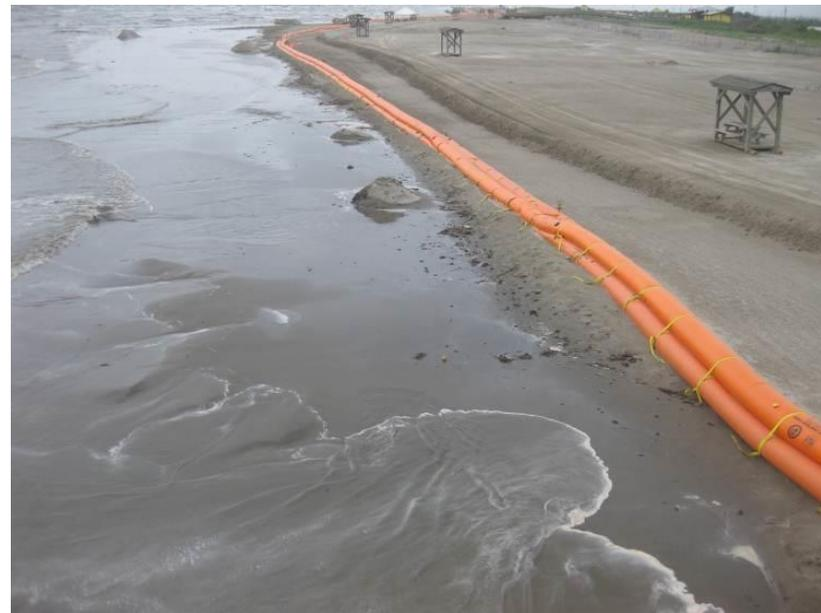
Water-ballasted boom anchored to form a barrier at the high water level. Note the low sand ridge on the landward side of the boom.
