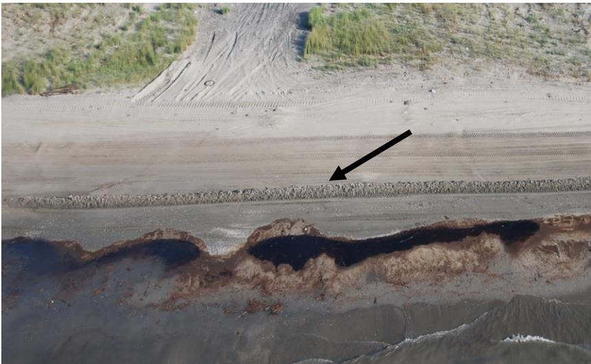
Aerial views of low (1-m) sand ridge being constructed by a road grader above the swash line as oil washes ashore.
